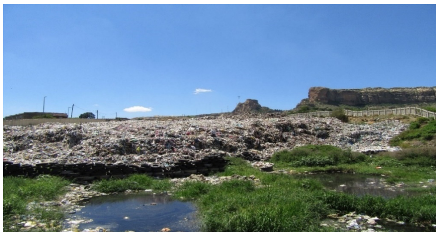
Figure 8: Leachate trickling from waste at the Tsosane landfill of the Maseru City Council.
